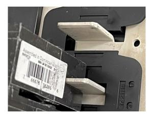
Tip: Align the breaker first and then seat the breaker in the load-center slot.
