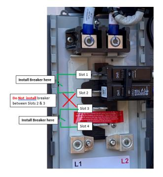
Example of where the breakers can be installed:
