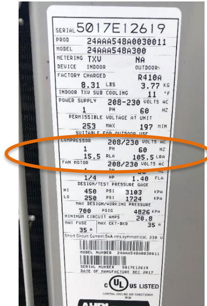
Figure 6: Example HVAC nameplate
