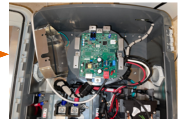
Figure 2b: E3 cover after being removed
