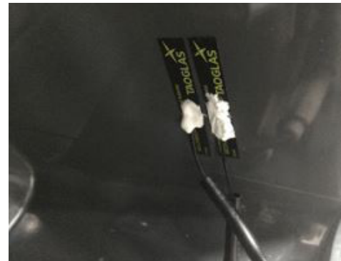
Figure 6: Pasting new Zigbee antenna adjacent to existing one
